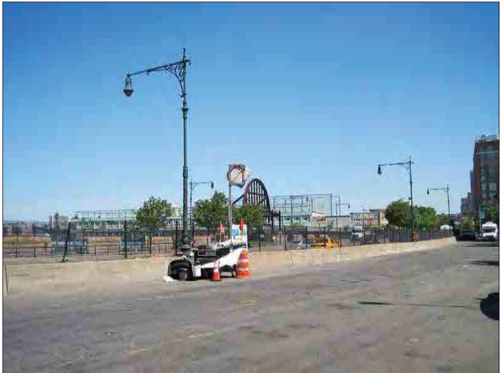
View northwest on West Street between Little West 12 th Street and Gansevoort Street 14
