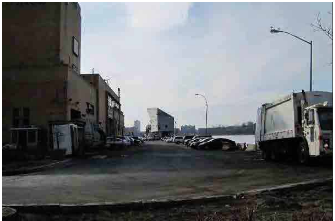
Pier 53: Marine Company One. View west from Hudson River Park 6
