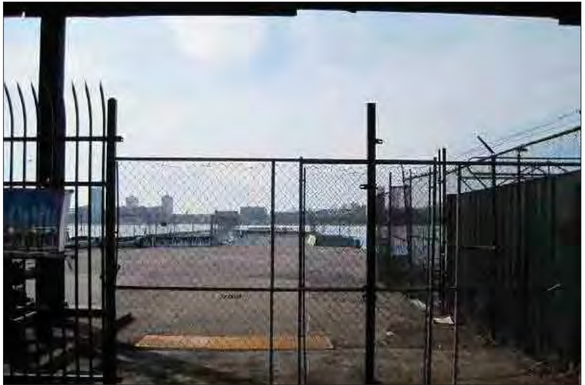
View west at existing Pier 54 1
