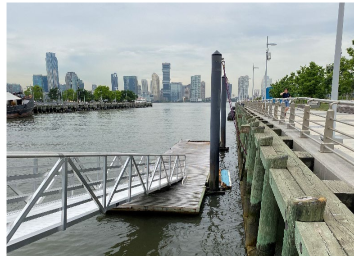
Fig. 2 | Pier 26 gangway and floating dock
