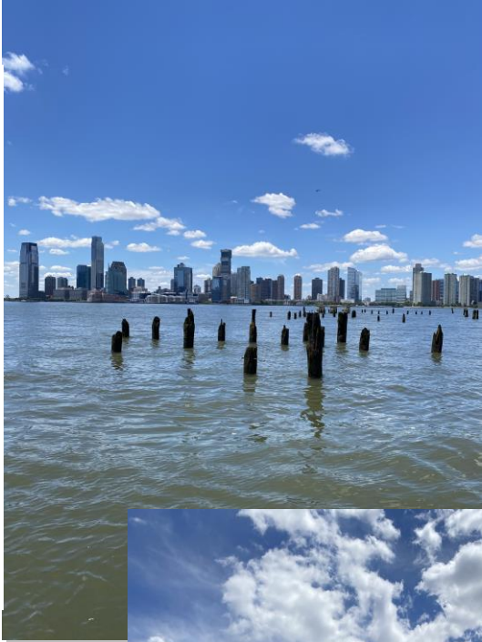
Fig. 7 | The Pier 32 pile field in which wraps are deployed.
