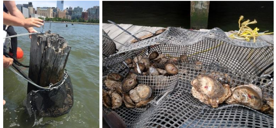
Fig. 2a (left) | Oyster wrap on a pile in deployment process. Fig. 2b (right) | Interior of an oyster wrap with oysters sitting on shelves in order to reduce crowding inside wraps.
